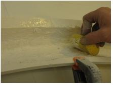
**10.** Once backing mud is dry, mix a small batch (1-2 ounces at a time) of gypsum cement powder with the add mix (DO NOT ADD FIBERGLASS TO THIS MIX!). Moisten the front (or face) of the joint and then fill the joint with this mud. Sand and repeat for 2-3 coats. (Note: You could also use quick-set drywall mud, or automotive Bondo if you prefer — used in pictures below.)
