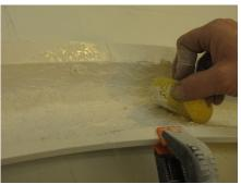
**10.** Once backing mud is dry, mix a small batch (1-2 ounces at a time) of gypsum cement powder with the add mix (DO NOT ADD FIBERGLASS TO THIS MIX!). Moisten the front (or face) of the joint and then fill the joint with this mud. Sand and repeat for 2-3 coats. (Note: You could also use quick-set drywall mud, or automotive Bondo if you prefer — used in pictures below.)
