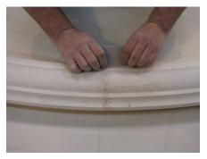
**11.** Our domes and light coves come with a paint grade finish (i.e. they are prepped for painting). For best results, lightly sand the entire surface after installation (to remove any hand oils, dirt, etc.), prime, and paint (water-based or oil-based primers and paints are fine).
